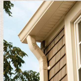
Rainware, Fascia, Soffit
